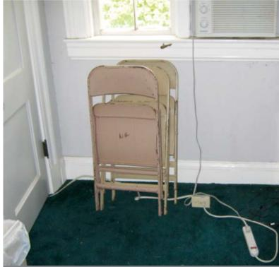
Bottom: This image shows several wiring hazards: a "homemade" extension cord on the floor runs under a doorway, which has an outlet installed at the end that has a power strip plugged into it that is supplying power to a window air conditioning unit. This is a fire just waiting to occur.
