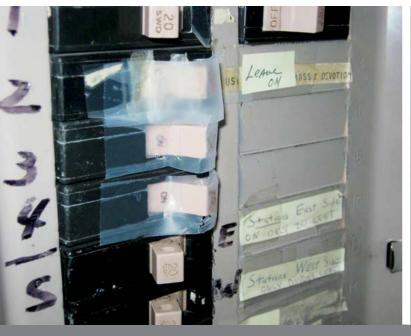
The image above shows breakers taped in the ON position. This practice should never be done.
