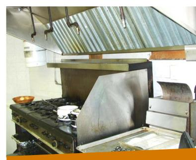
This photo illustrates the correct installation of a metal baffle plate between the open flames from the range and the deep fat fryer. Metal baffles should be used only when there is not sufficient space available to provide a 16-inch clearance between the deep fat fryer and any source of open flames.
