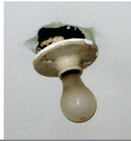
Bottom left: This image shows a broken light fixture. This exposes the wiring to physical damage, dust, dirt and moisture accumulation.
