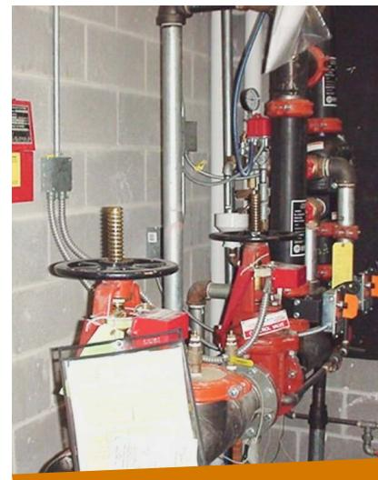
This photo shows an example of a sprinkler system main valve. Note the inspection repor attached to the sprinkler main. The report contains information on the sprinkler system, when it was last inspected and details regarding the inspection.
