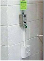
These photos are examples of manual activators that should be used if the automatic extinguishing system fails to activate. Such devices should be installed away from the cooking surface, next to an entrance/exit for the kitchen. Kitchen staff should be aware of this manual activator and trained on its use. Also note the inspection tag. Many fire service companies place these tags on the manual activator to indicate current servicing.
